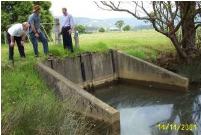
Normal floodgate opening to Broughton Creek.
