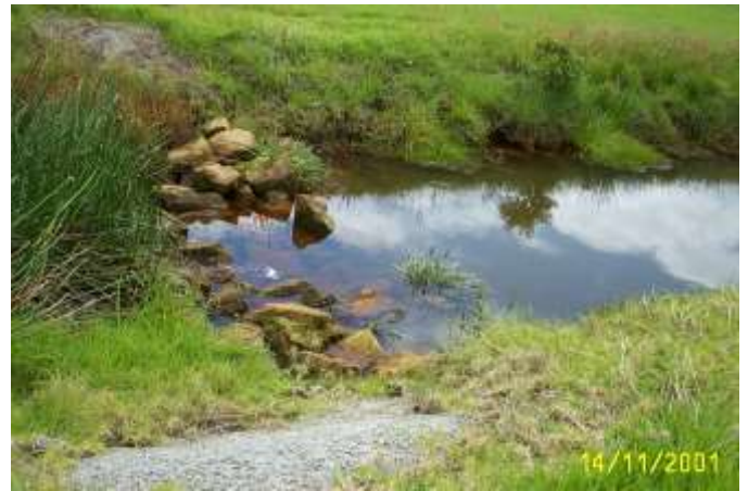
Weir constructed by UOW to raise water level. Saline water to right of weir stops growth.
